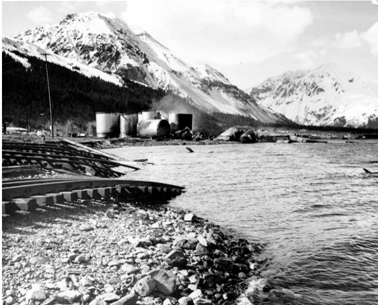
Seward was damaged by shaking from the earthquake and then the tsunami. The earthquake caused significant subsidence and failure of the waterfront. Here the rail track can be seen diving into the slumped ground. View of damage to waterfront, Seward, Alaska, after March 27, 1964 earthquake. March 1964. Photographer: U.S. Army (Alaska Digital Archives)
