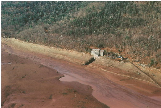
Figure 1: Aerial view of sediment below 1065' immediately in front of the Shandaken Tunnel Gatehouse. Photo courtesy D. Wood, c. 1993
