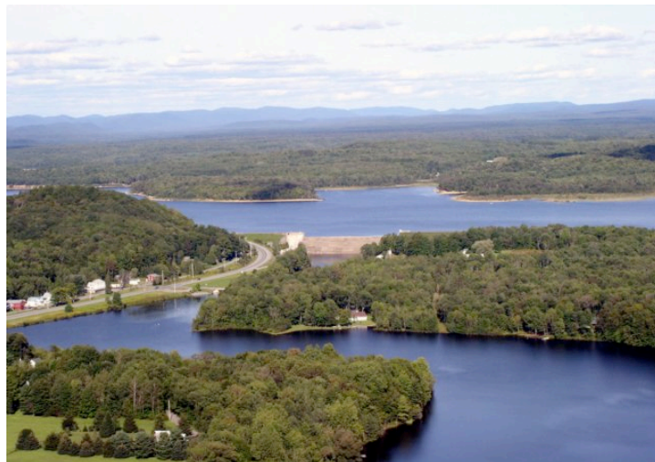
Figure 4: Dammed Hinckley Reservoir in the background and Prospect Reservoir below the dam in the foreground (Ram-Air Skyways, 2006).
