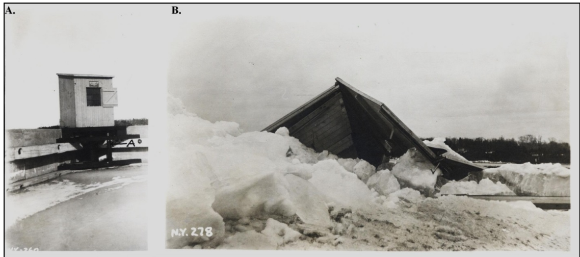
Figure 3. U.S. Geological Survey station no. 01356000 – Mohawk River at Vischer's Ferry Dam, NY: (A) before flood of 1914; (B) after flood of 1914 (March 28, 1914).
