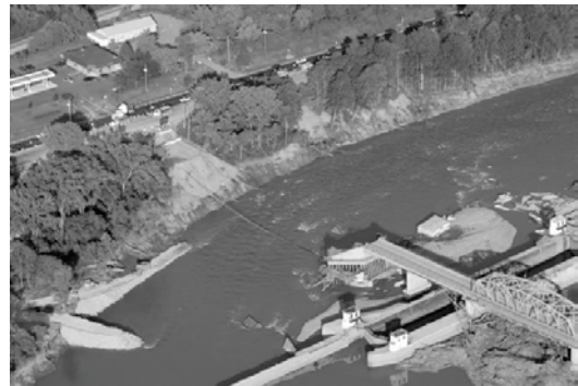
Figure 2. New York State Route 103, adjacent to Lock E-9 in Rotterdam Junction, was washed away following Hurricane Lee.
