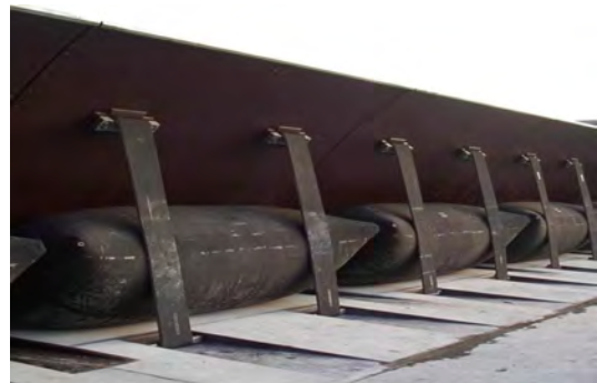
Obermeyer gate structure showing inflatable bladders.
