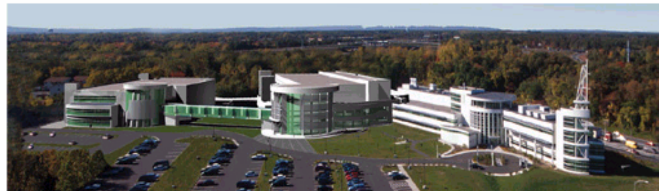
Albany NanoTech complex with Business Incubator/Technology Accelerator on left, 300 mm wafer R&D fab in center (both under construction) and existing 200mm wafer R&D facility on right.
