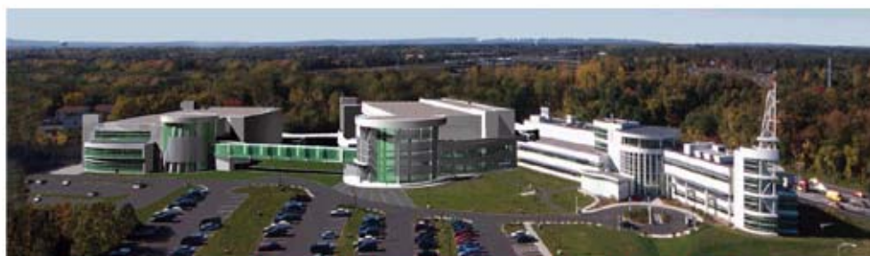
Albany NanoTech complex with Business Incubator/Technology Accelerator on left, 300 mm wafer R&D fab in center (both under construction) and existing 200mm wafer R&D facility on right.
