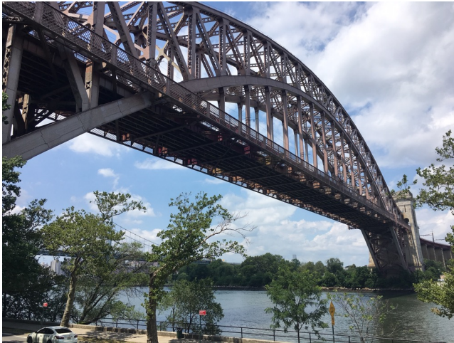
Hell Gate Bridge in Astoria Queens. Photo: SM LaBrake
